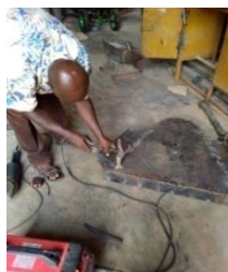
Plate 3a: welding a galvanized pipe for water passage
